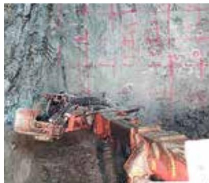
Face being drilled with the paint lines as a guide.
