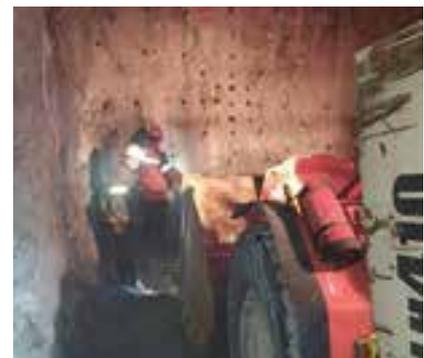
Face after drilling, being charged with explosives.
