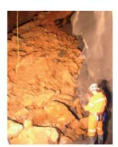
Face collapse, weathered sands/clays, with no cohesion and no strength
