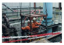
Fig. 9 — Workers access the Fresh Air Shaft to assist with the removal of the Alimak Emergency Exit equipment from the Mine.
