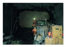
**Fig. 15** – Employees work on the installation of the barricade at the base of the plug on the decline.
