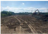
Fig. 18 – The completed decline / portal plug – covered over with overburden.
