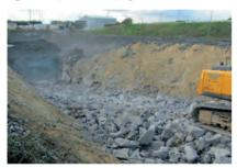
*Fig.* 17 – Work to seal the portal section on top of the decline plug on the decline.
