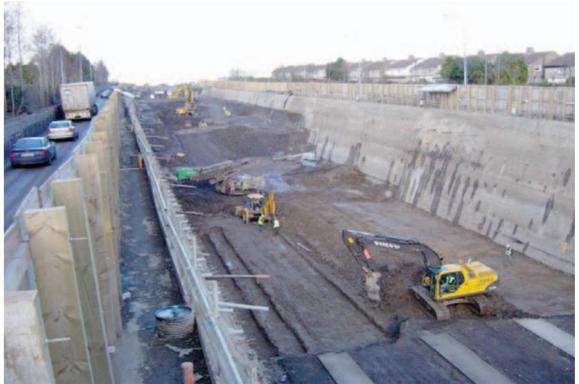
Figure 1. The 'Cut & Cover' Tunnel Excavation.
