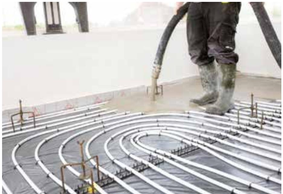
selection and use of screed materials provides physical and performance requirements and definitions for factory produced materials. It is referenced in this context by BS8204.
