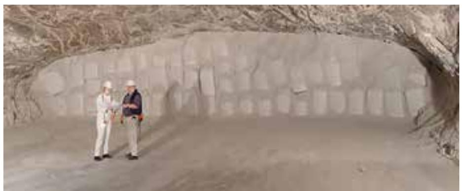
German Salt Mine – Solidified & Bagged APCr Structure at an Underground APCr Recovery Facility
