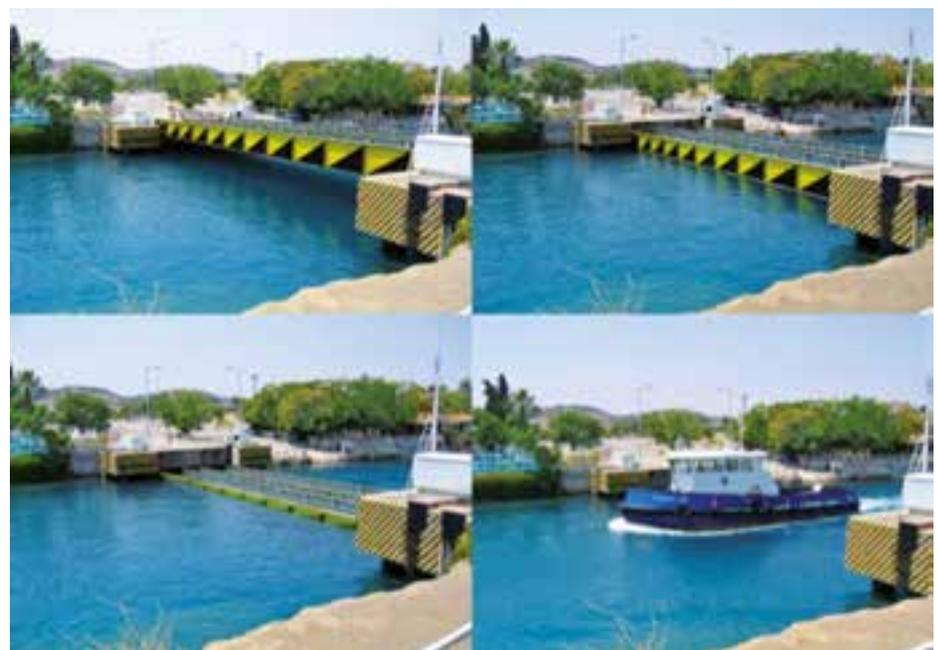
A bridge being submerged to allow boats to pass through.
