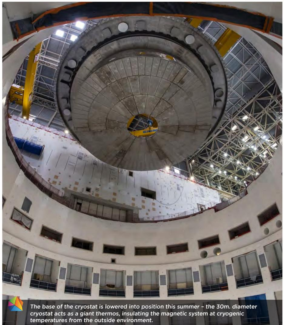
The base of the cryostat is lowered into position this summer – the 30m. diameter cryostat acts as a giant thermos, insulating the magnetic system at cryogenic temperatures from the outside environment.
